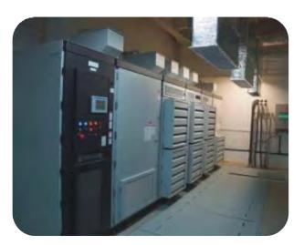
Additional reason to choose this frequency converter was the necessity to provide continuous unit operation for 4 year period of time.
