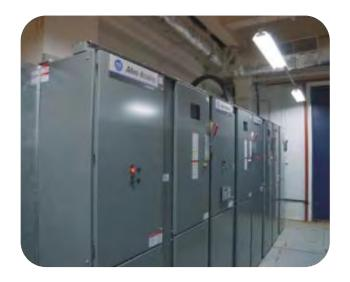
Start-up and adjustment work, including by-pass switch check were performed within 8 days by Rockwell Automation staff with the help of «BPA» Company.
